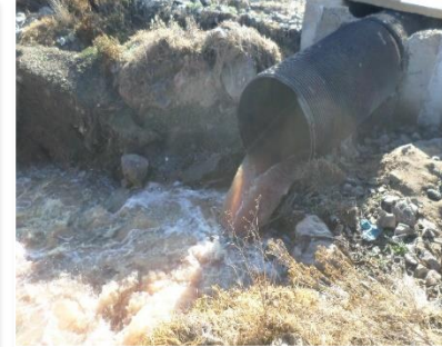
Mangaung (FS): Untreated effluent flowing directly into environment (Botshabelo WWTW)
